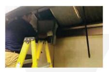
Grip the handles firmly to safely remove the filter from the hood.
