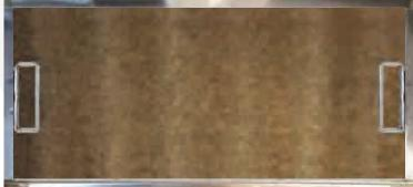
Filters are starting to show grease accumulation. Notice the "ribs" of the baffle filter becoming visible.
