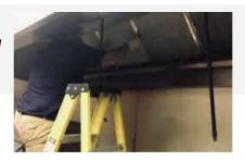
Using the handles, place the filter back into your system. Make sure the handles are on the sides (not top/bottom).
