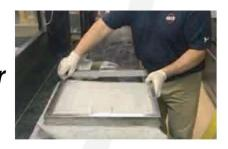
Place a new filter on top of the frame and then "snap" the cover in place by lining up the nipples and dimples on the sides of the filter.
